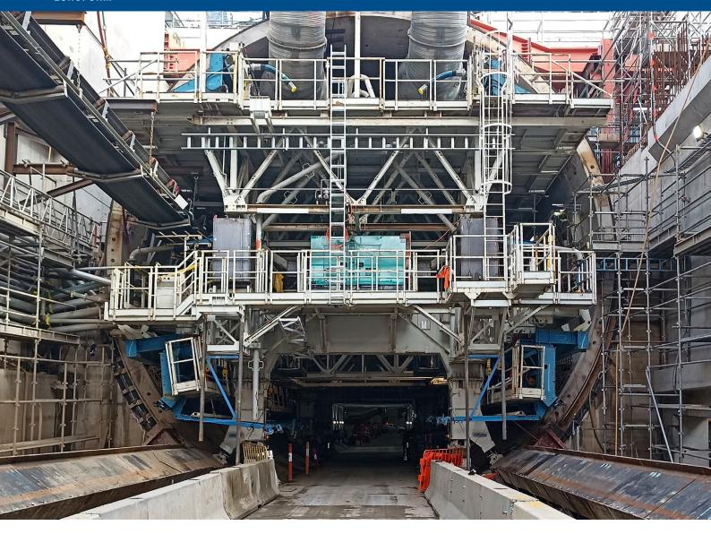
HIGH-TECH CONVENTIONAL FORMWORKS AND SEGMENT MOULDS FOR PRECISE TUNNEL LINING
