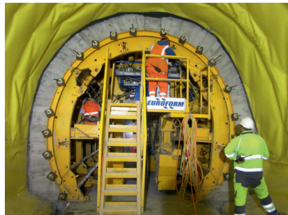
Cross passage formwork
