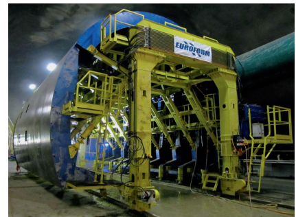
Collar formwork
