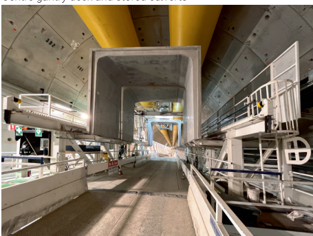
Centre gantry deck and stored culverts
